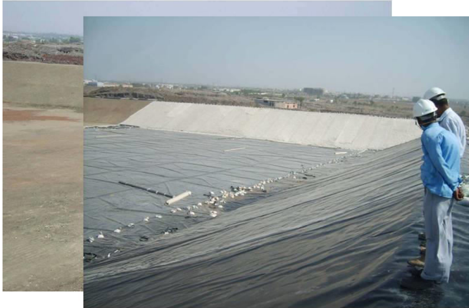
Liner Installation
